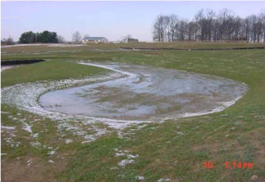
During site development, efforts are made to protect soils and prevent compaction of soils in future infiltration trenches (here a chain link-filter fabric baffle helps to control sedimentation). When construction is complete, soils will be scraped and percolation tests will be performed to ensure soils permit infiltration.
