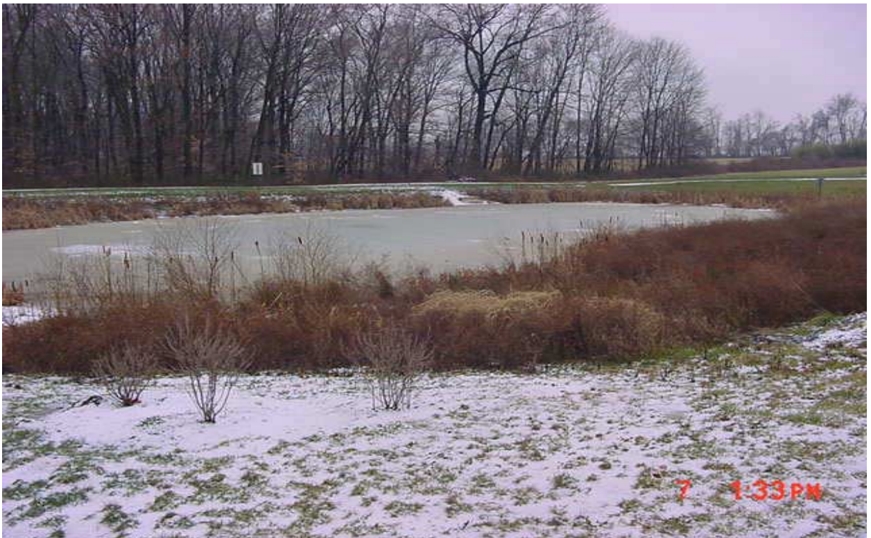
This constructed wetland maintains wet pond year-round. Wetland plantings stabilize banks through the winter.
