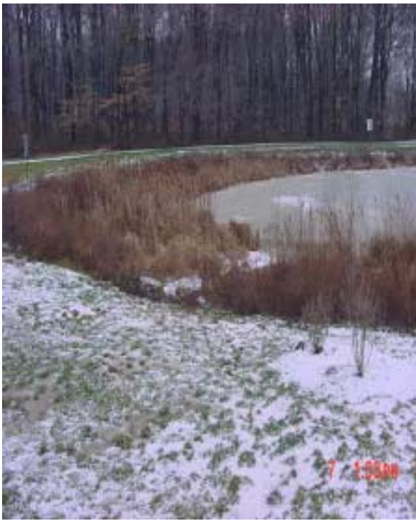
This constructed wetland maintains wet pond year-round. Wetland plantings stabilize banks through the winter.
