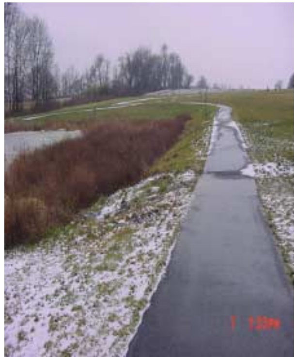
This constructed wetland maintains wet pond year-round. Wetland plantings stabilize banks through the winter.
