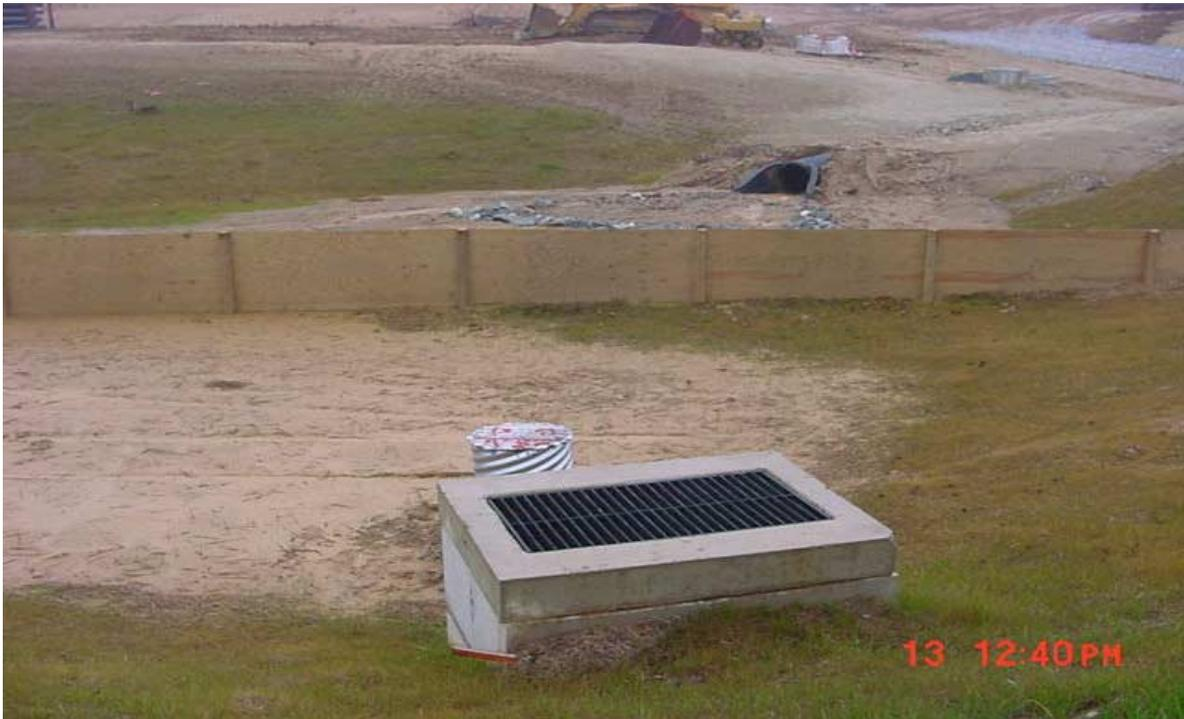
During site construction measures are needed to prevent compaction of soils by equipment and excessive sedimentation since this structure will be converted to an infiltration basin when construction is complete.
