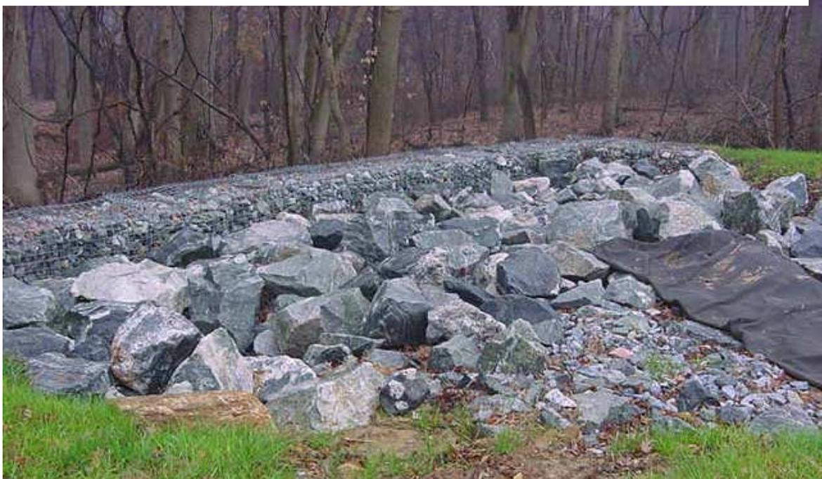
Rock and level spreader (riprap contained in wire cages) pictured in the middle of picture used during construction to dissipate energy and disperse stormwater discharging basin into the adjacent wetland.
