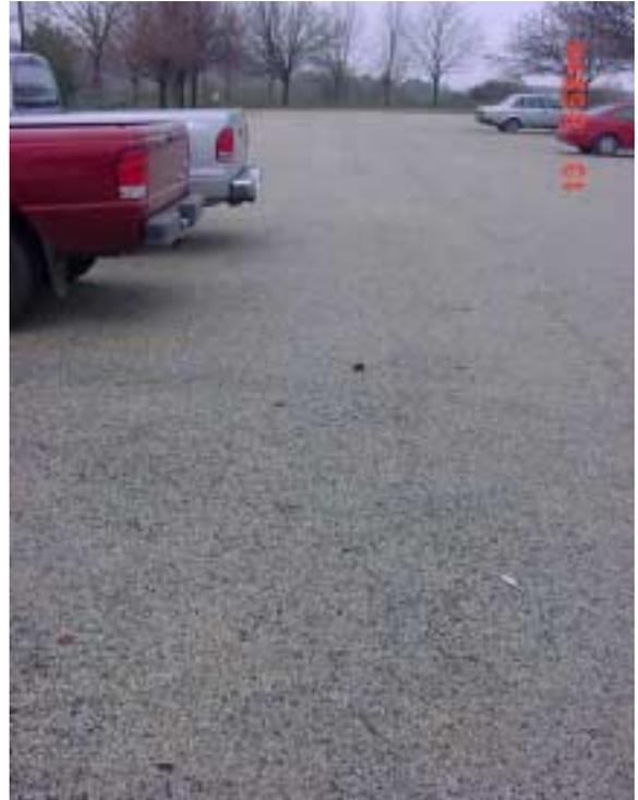
To limit compaction, porous pavement lot used for passenger vehicle parking only.
