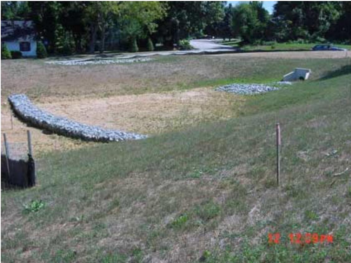
This photo shows the riprap berm in the basin that separates the forebay from the adjacent detention basin. Entering stormwater flows into the sediment forebay first before flowing through the riprap berm into the adjacent basin.
