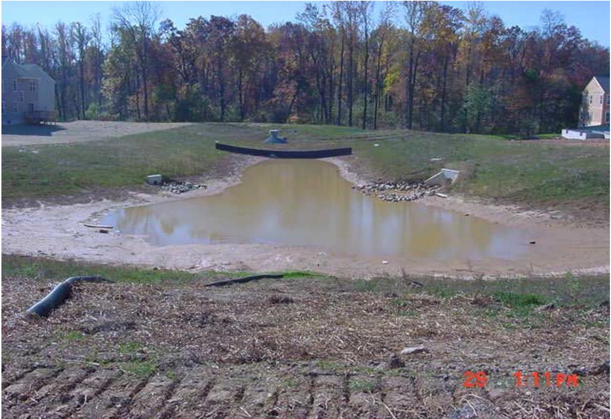
During site construction measures must be taken to prevent soil compaction that can result from heavy equipment and excessive sedimentation. When site construction is complete, soils will be tested to verify their permeability and ensure infiltration.
