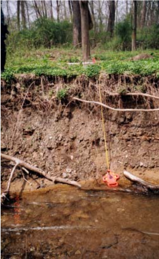
Exposed, vertical banks are found throughout the watershed, allowing instream erosion to mobilize and transport soils from the stream banks.
