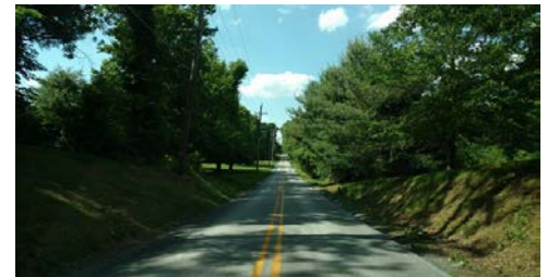
The 1728 Road of the Great Valley, modern Northbrook Rd. looking north. The 18 th century roadbed and alignment is still evident with the deeply incised road banks and still relatively narrow cartway.
