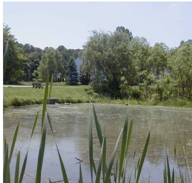
Stormwater retention basin (pond) integrates access for pedestrians as well as providing vegetation along the shoreline.
