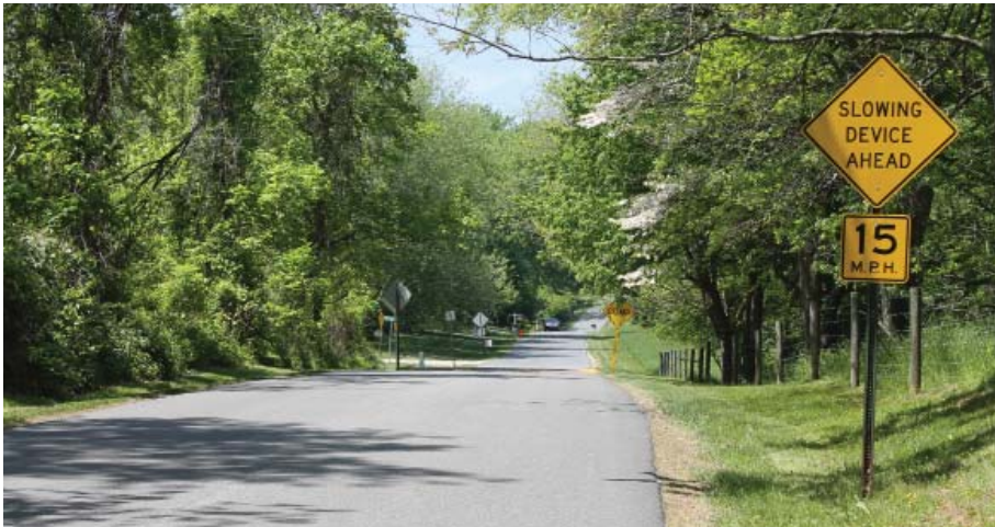
Traffic calming measures.
