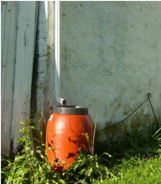
Rain barrels capture roof runoff. With a soaker hose attached, this BMP can also help your garden survive drier periods.
