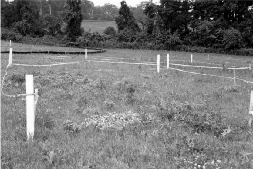
**Primary and replacement absorption areas in an open space area. They have been staked, surveyed, and cordoned off so the area is not disturbed until the system is installed.**
